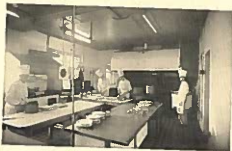
Typical of behind the scenes showing a section of our model hygienic Kitchens with latest stainless steel equipment, tiled walls and modern lighting.
